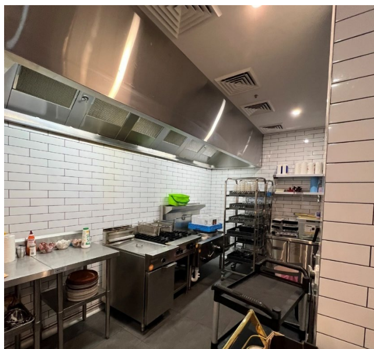
Figure 40 Industrial kitchen at 94 Hay Street.
